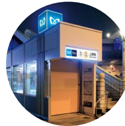
Building disaster resilience
