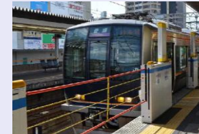
Platform Screen Door
