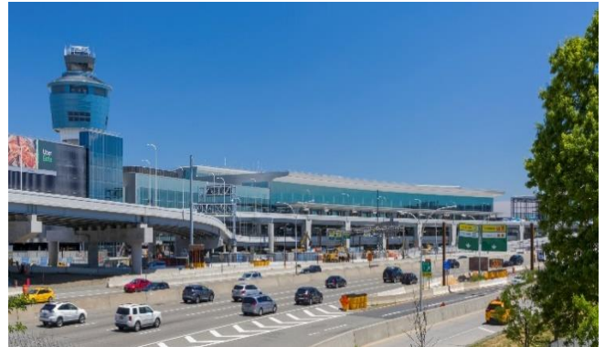
Figure 5. Exterior View of LaGuardia Airport Terminal B
