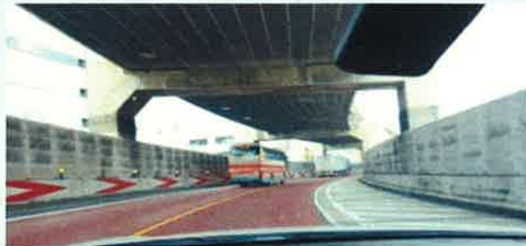
Double deck (GPS reception issues)
