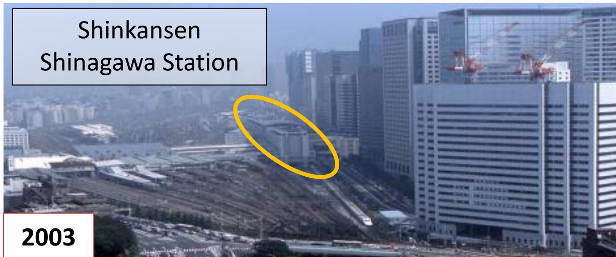
When Shinagawa Station was put in place
