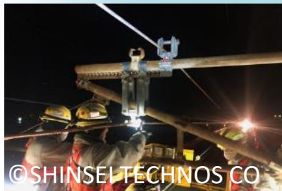
Construction & maintenance works
