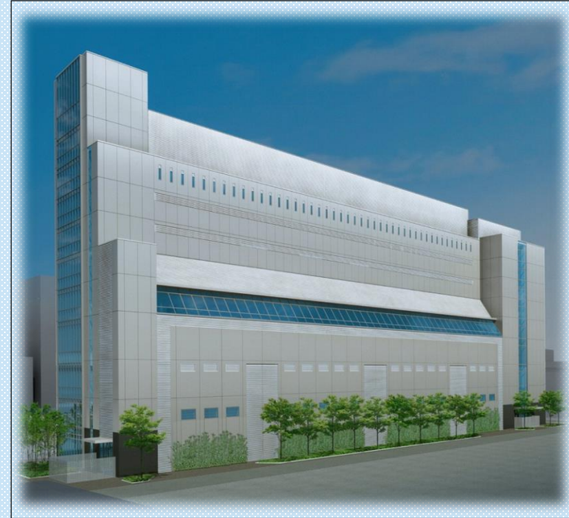
Southeast-side exterior (main entrance side)
