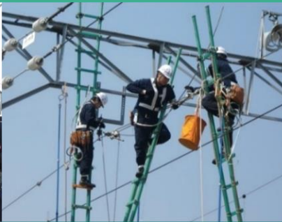
Training for repairing catenary
